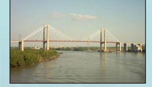
All of the deck support cables lead directly back to the supporting columns.
